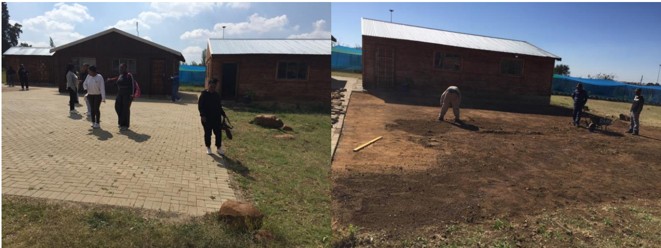
The before-and-now of the land scaping and paving in progress
